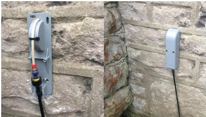
This is the box that is attached to the outside of your house that guides the fibre optic cable into your home.
